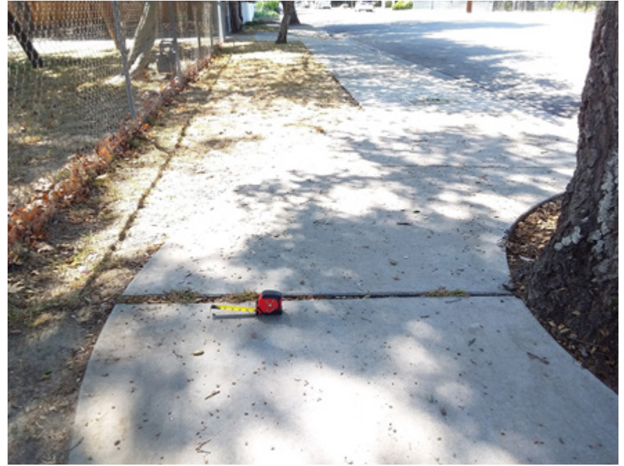
FIGURE 2-9: Horizontal separation
