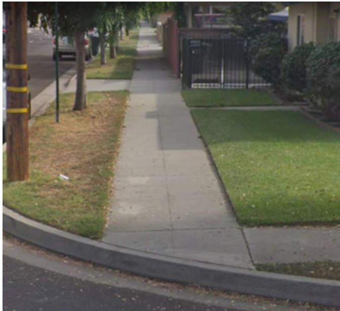
No curb ramp, street view
