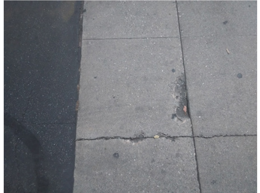
FIGURE 2-7: Spalling
