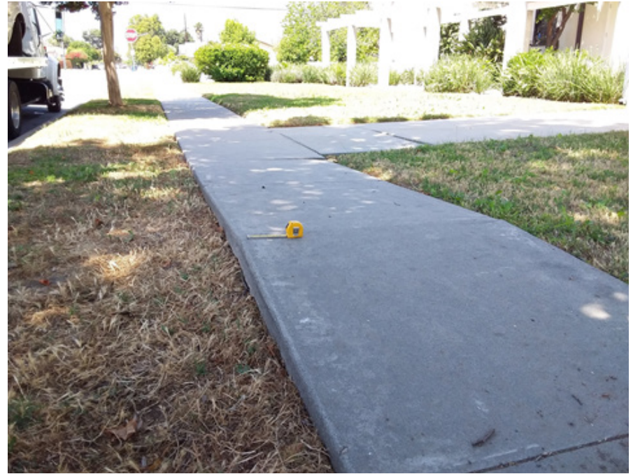
FIGURE 2-5: Sidewalk hump
