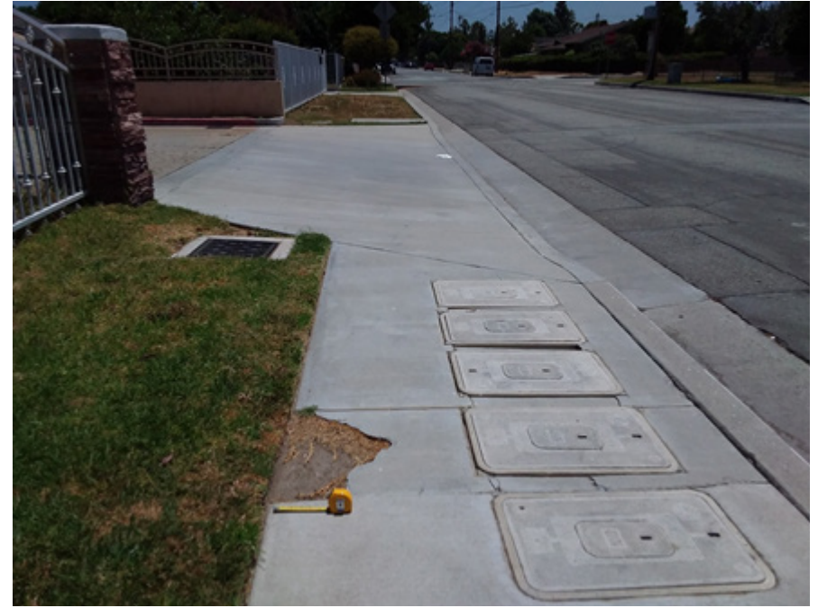
FIGURE 2-11: Broken panel
