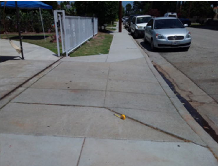
FIGURE 2-3: Driveway approach in scope
