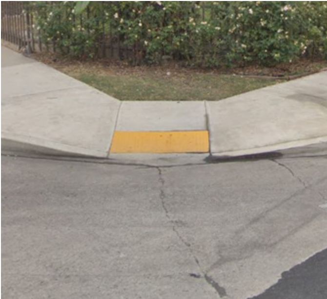
Visually compliant curb ramp, street view
