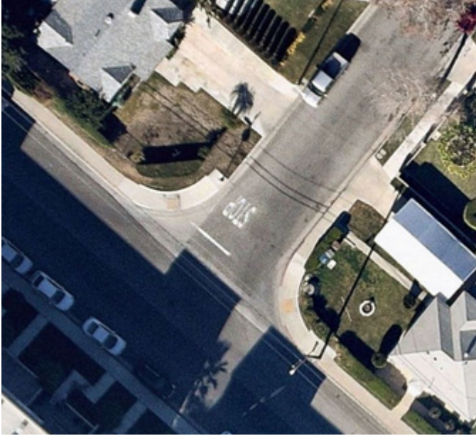
Visually compliant curb ramp, aerial view
