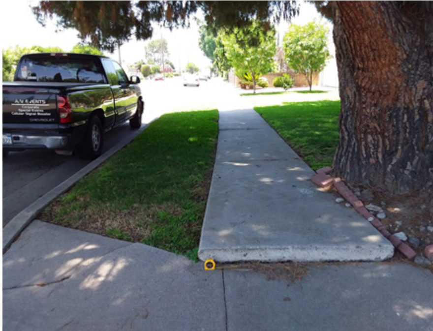
FIGURE 2-12: Vertical separation
