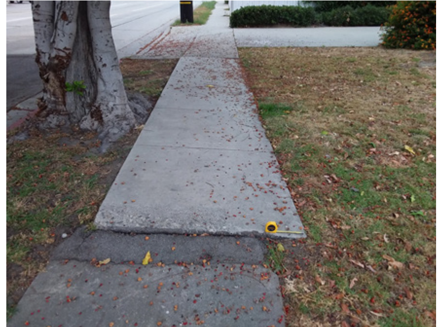
FIGURE 2-13: Horizontal displacement
