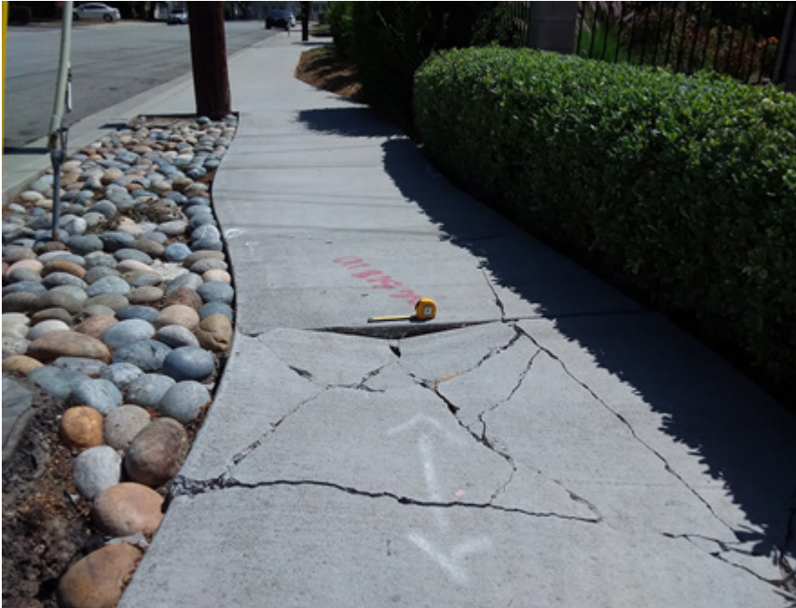
FIGURE 2-6: Sunken sidewalk
