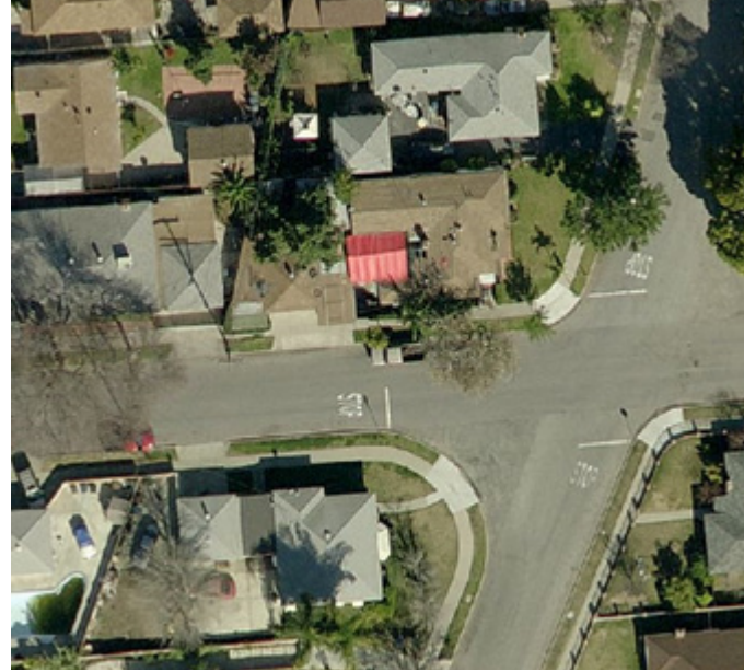
Visually non-compliant curb ramp, aerial view
