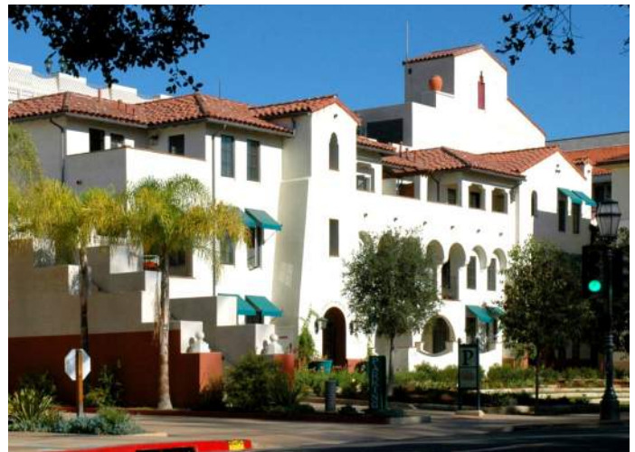
Variety of material and colors in a mixed-use building.
