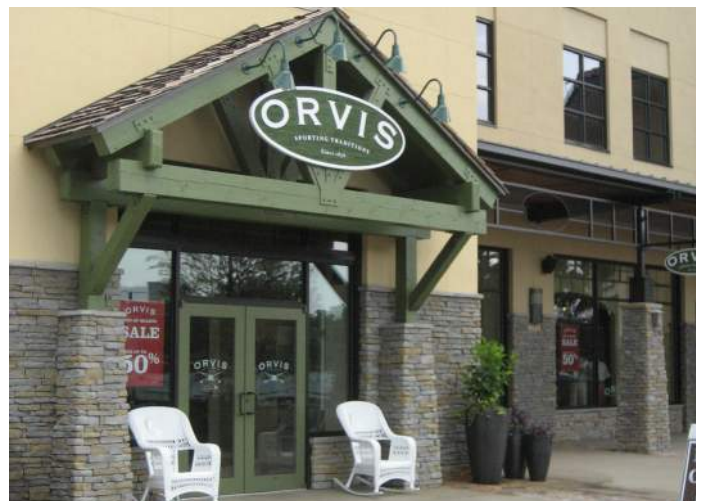
Prominent building entry.
