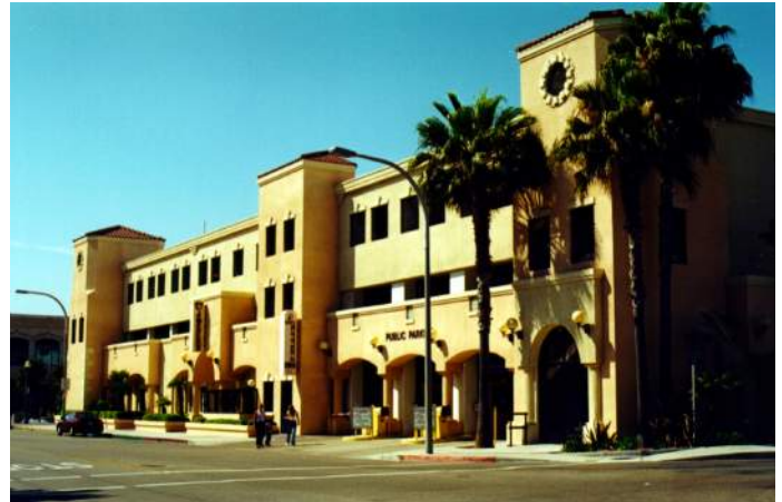
Parking structure facade is broken up with variation in massing.
