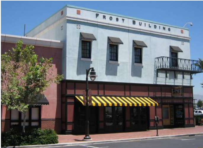
Awnings located over doors and windows.
