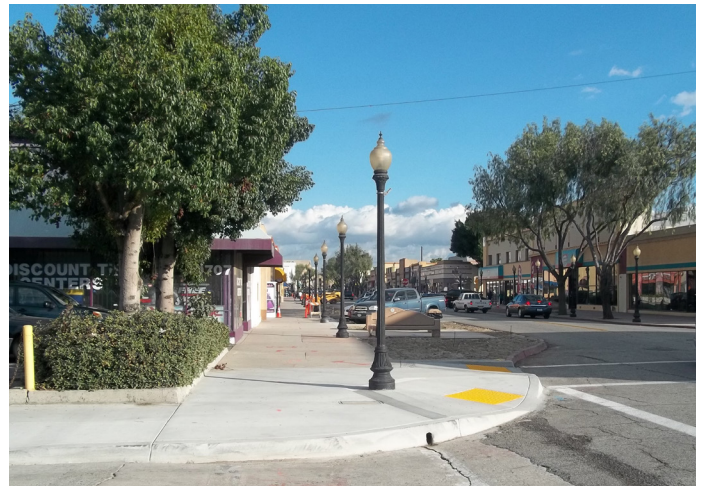
Existing Pedestrian Lights along Main Street.
