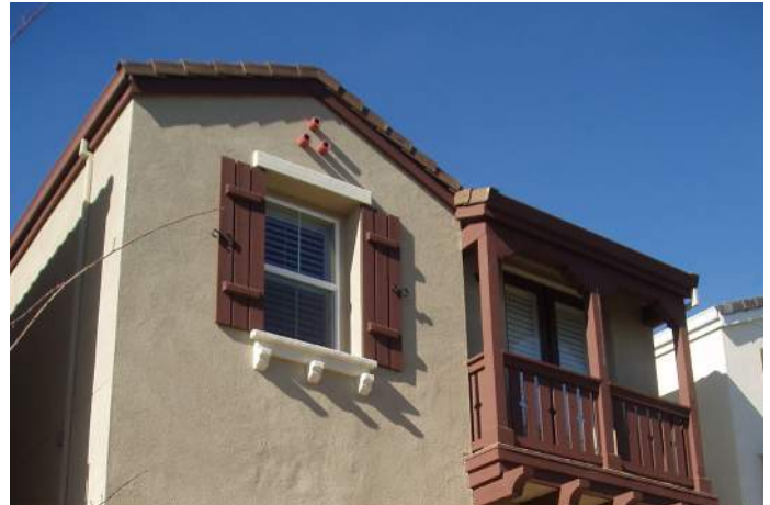
Windows articulated with proportional shutters.
