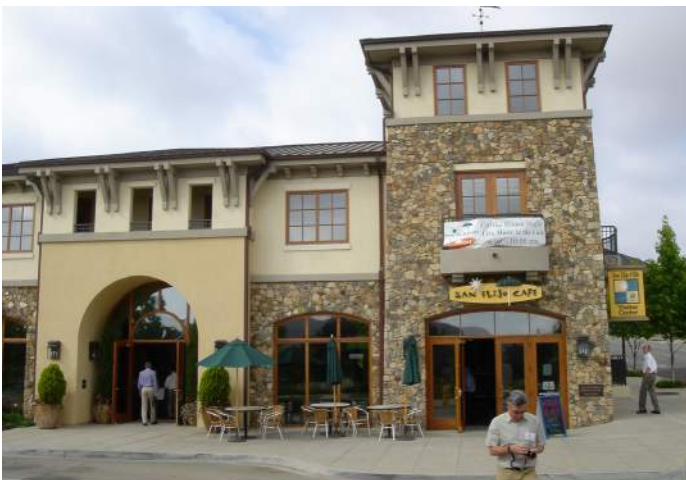
Deep roof overhang with exposed structural elements.
